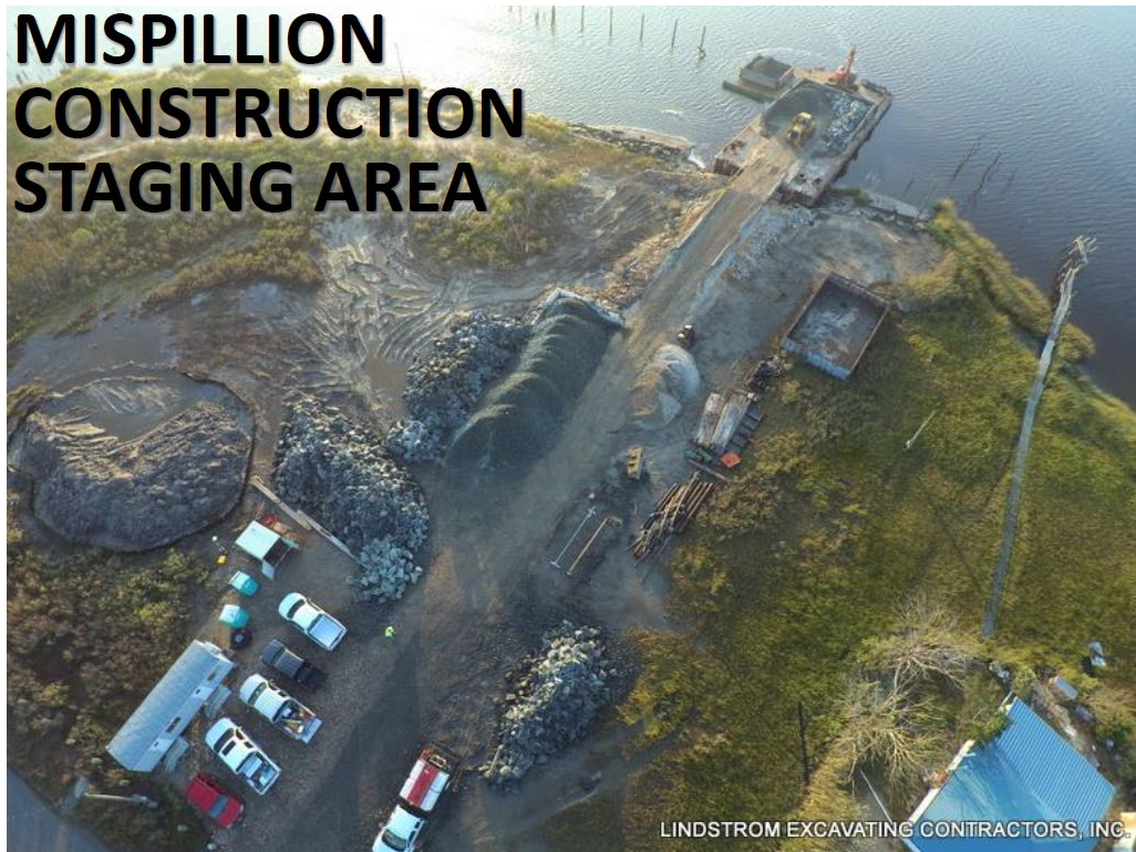
Figure 4-8. Photo of Staging Area in 2018 (Moffatt & Nichol, 2018)
