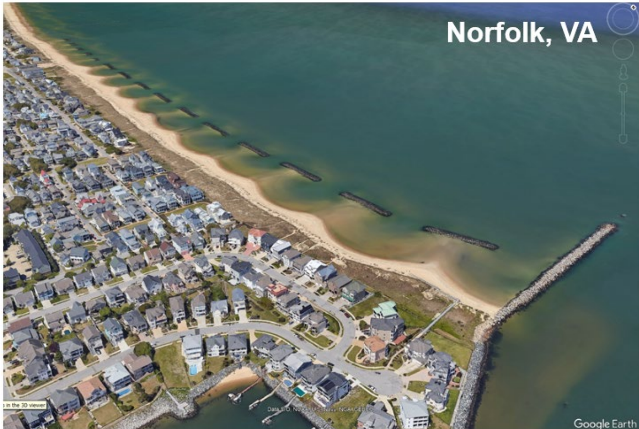
Figure 4-6. Example of Nearshore Breakwaters at Norfolk, VA
