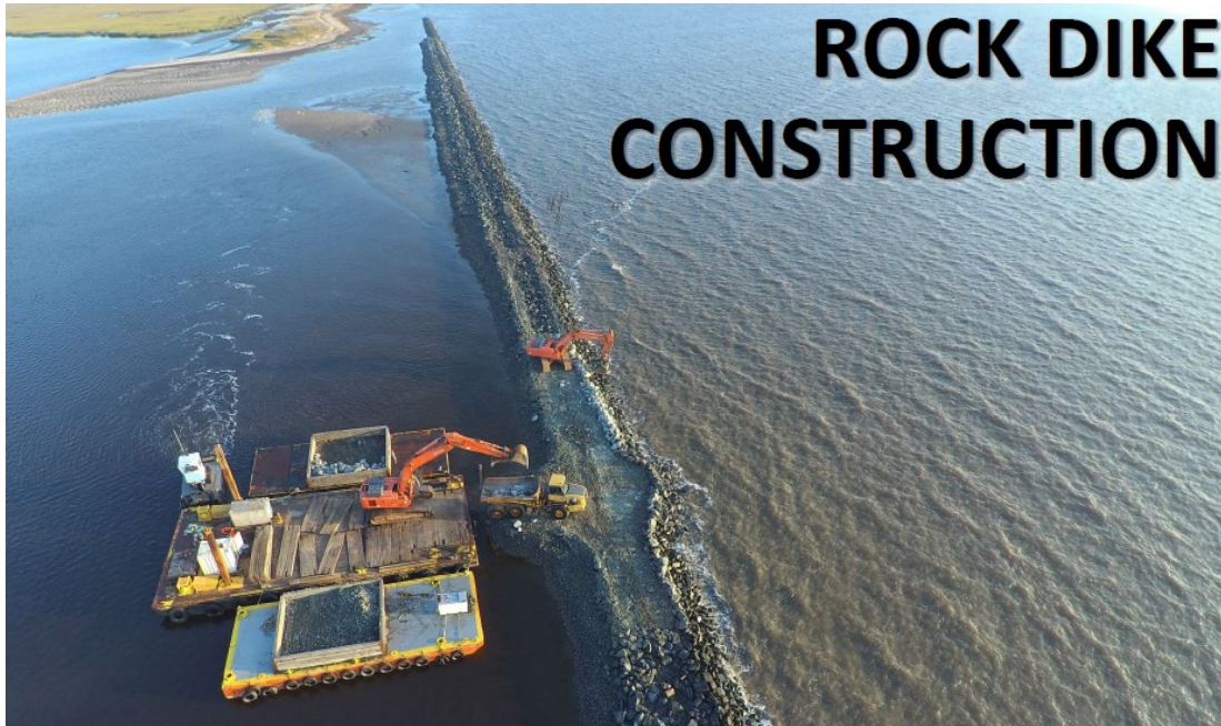
Figure 4-7. Photo of Dike Construction in 2018 (Moffatt & Nichol, 2018)
